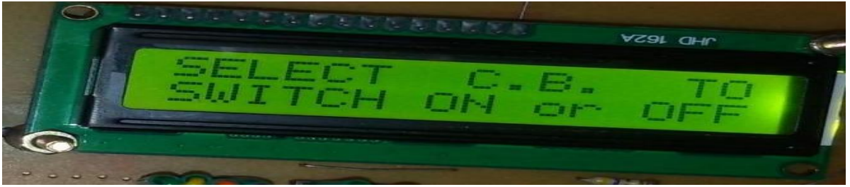
FIG. 5: IF THE CORRECT CARD IS GIVEN THEN IT WILL SHOW THE SELECT THE CIRCUIT BREAKER TO BE OFF
